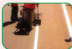
Road Maintenance Coatings
